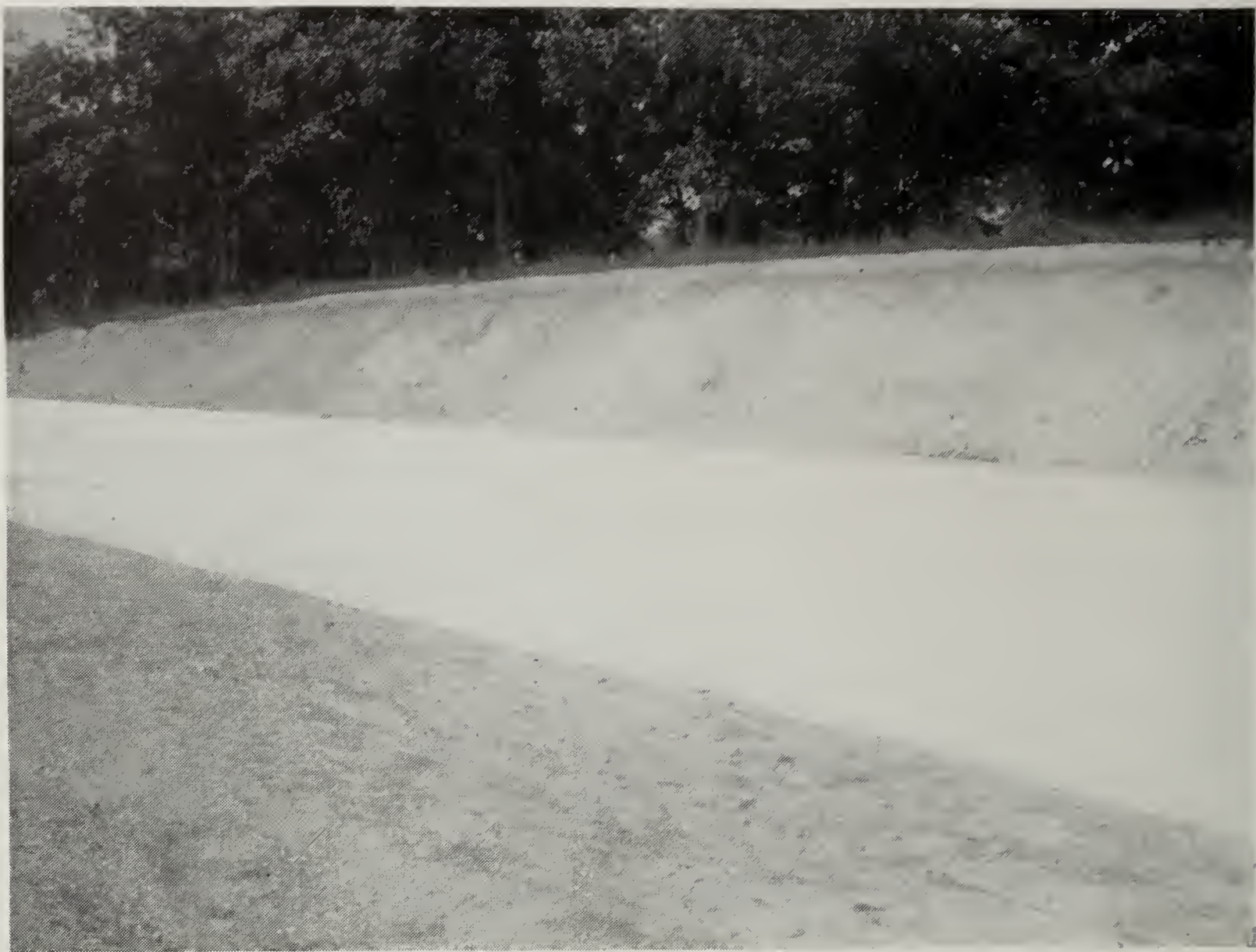
FIG. 7.—Road cut along Southwest Highway at Worth showing soil profile typical of the Chicago region. The uppermost zone of a few inches is ash-colored (forest soil) and has lost its lime and most of its iron. The underlying dark zone is reddish colored owing to a concentration of iron oxide. Below the rusty iron oxide zone is gray unweathered glacial till in about the same condition as at the time of its deposition.
